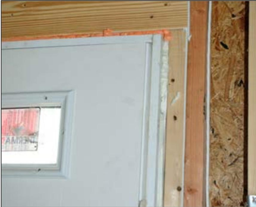
Gaps between framing and windows or doors shall be sealed with minimally expansive foam.
