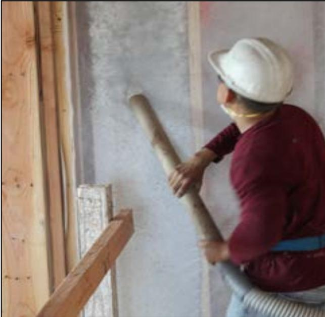
Loose fill insulation includes loose fibers or fiber pellets that are blown into building cavities or attics using special equipment. Typical loose fill insulation products include mineral fiber (fiberglass or rock-wool) or cellulose. They are installed in walls, floors, attics and below roofs using a dry-pack process or a moist-spray technique. They may include a netting material for support.
