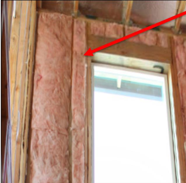
Non-standard width cavities shall be filled with insulation to snugly fit into the space, or with minimally expansive foam sealing material.
