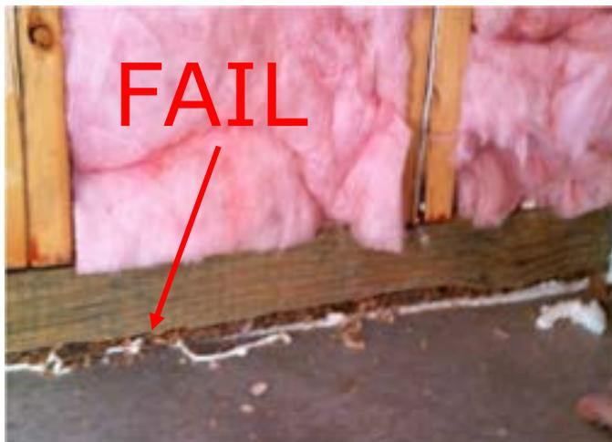
This photo shows a poor job of spray foam being used to seal the bottom plate on a slab on grade application. This is not acceptable and would fail QII.
