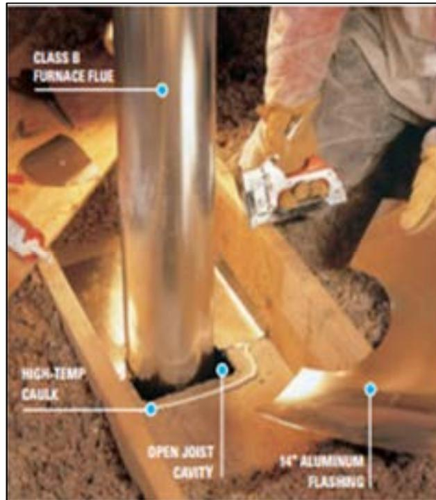
Once the base flashing is cut, sealed and secure, high temperature caulking is used to seal between the flue pipe and the base flashing.
