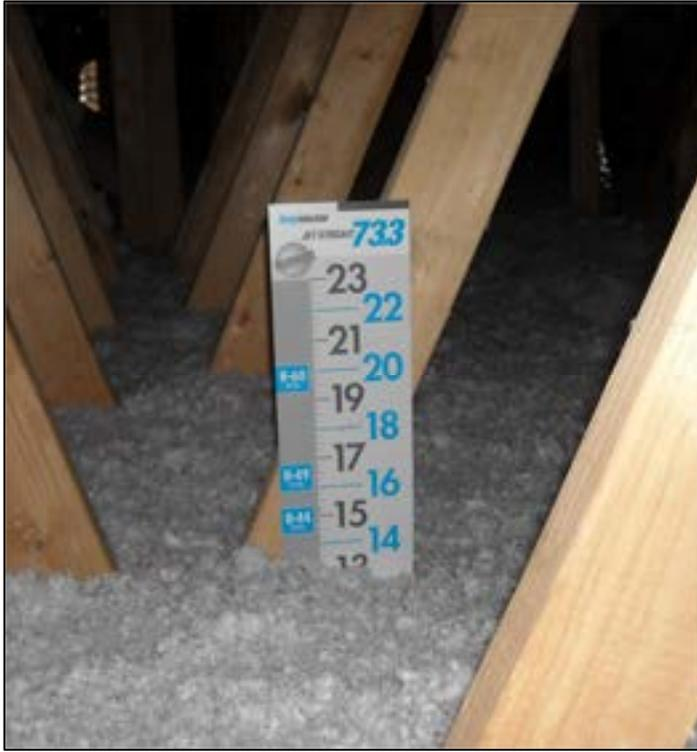
Attic rulers appropriate to the material shall be installed and evenly distributed throughout the attic to verify depth: one ruler for every 250 square feet and clearly readable from the attic access.
