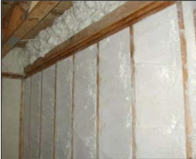
Spray polyurethane foam is a two-part liquid foamed plastic material formed by the reaction of an isocyanurate and a polyol. This application uses a blowing agent to develop a cellular structure when spray applied onto a substrate. SPF insulation can be formulated to have specific density, compressive strength, fire resistance and R-value.
