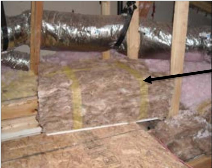
Attic access cover insulated with fiberglass batt. Notice the straps holding insulation in place.
