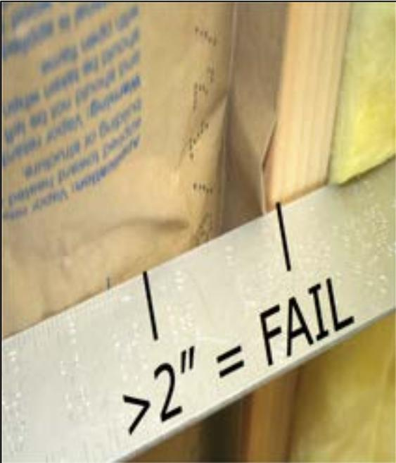
**Note:** Voids created by the flange inset which do not extend more than two inches from the stud on each side shall be allowed.
