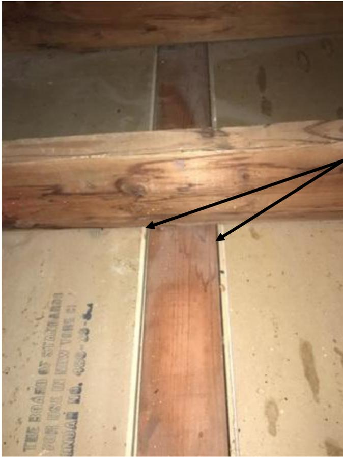
Another option to seal the top plate of all interior or exterior walls, the top plates would need to be sealed after drywall was installed. Air sealing would occur from the attic side typically using spray foam or caulking.
