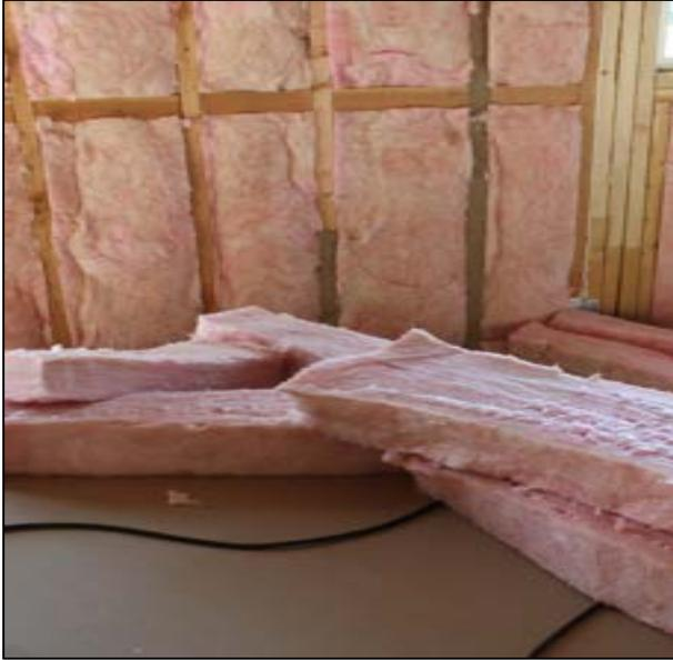
Batt and blanket insulation are made of mineral fiber and mineral wool, either:
