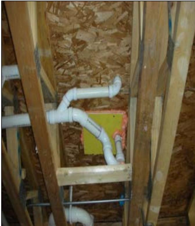
Plumbing access holes cut into the subfloor to set tubs and showers shall be sealed with a hard cover and caulk or spray foam.
