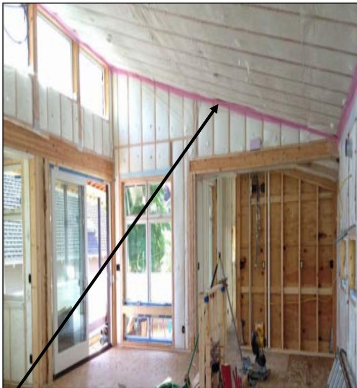
**CAUTION:** It has been recognized that drywall installers tend to remove this type of air sealing product as it may slightly interfere with installing drywall to the ceiling. Installers and builders should ensure this is left as is after an inspection. This could lead to multiple small leaks along the top plate of all interior and exterior walls.
