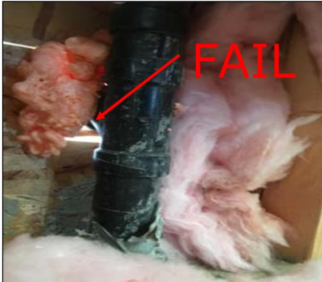
The photo shows a plumbing waste line clean out penetrating the exterior OSB. Spray foam was used to seal the gaps but much of it was missed. This is not acceptable and would fail QII.
