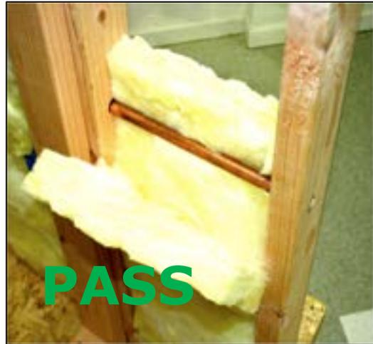
For example, a plumbing pipe located one-third of the distance from the front of the cavity should have batt insulation delaminated so that two-thirds of the batt is installed towards the outside wall surface and one-third is installed towards the inside wall surface from the pipe.
