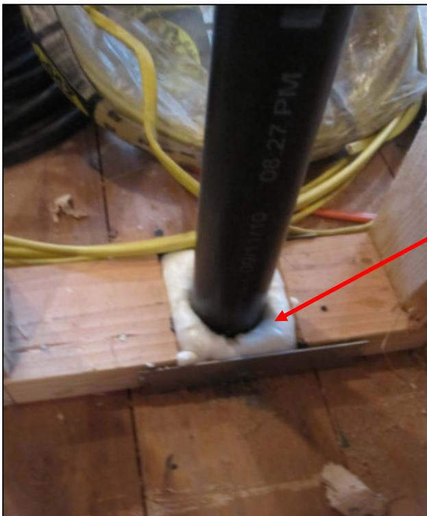
All plumbing, wiring or other penetrations through the subfloor and bottom plates, into the crawlspace or between floors shall be sealed with caulking or spray foam.
