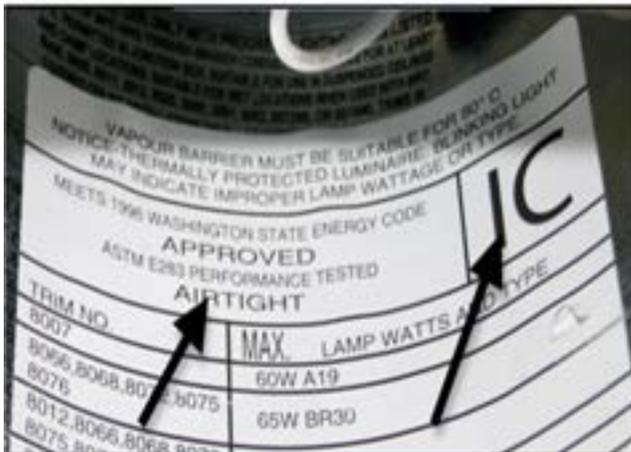
Raters need to also ensure that the recessed can lights are rated for insulation contact and are air tight (IC/AT rated).
