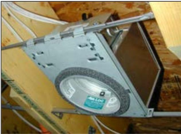
Can lighting typically comes with a foam gasket for sealing the can light to the drywall. Raters must ensure that these are present. If they are not present then caulking or spray foam is adequate.
