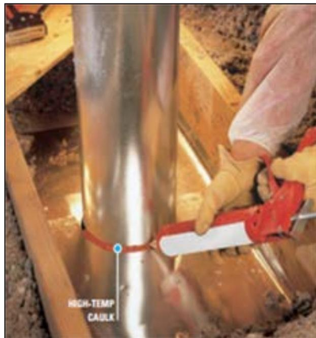
Lastly, a sheet metal dam is fabricated to wrap the flue pipe. Tabs are bent in at the top of the dam to help maintain the 1-inch clearance between the flue pipe and the sheet metal as insulation will be in contact with the sheet metal. At the bottom, tabs are bent out in order to secure the dam to the base flashing. The dam height needs to be high enough to be above the depth of the insulation required.
